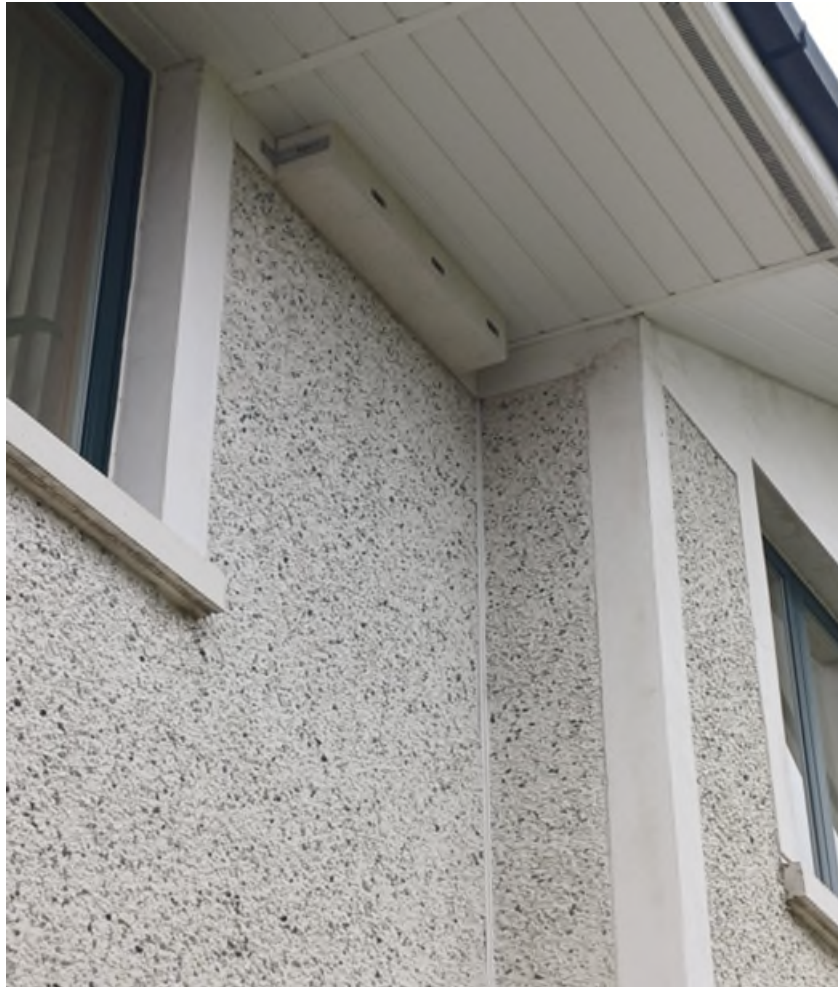
Above: Newly installed swift boxes on the Department of Education Campus, Tullamore.
